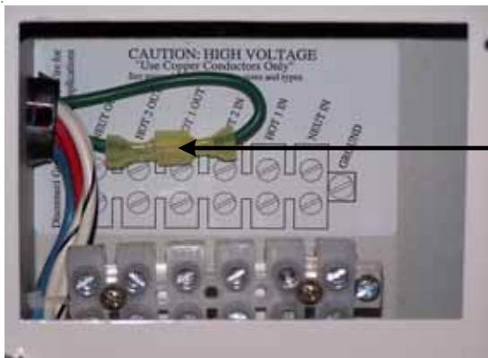
Figure 11, AC Wiring Compartment (MS models)
